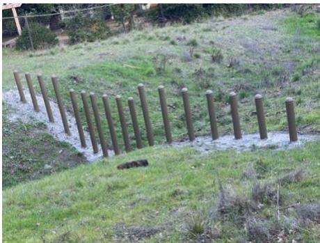
Heavy rain events mobilized off-site debris into several storm drains, causing blockages and flooding. The Deer Meadow Drive Storm Debris Catchment Improvement will consist of a series of upstream debris catchments.
